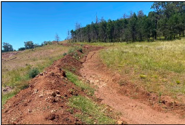
PHOTOGRAPH 2.3 (above): Earthen bund above Bolgers Pit diverts 'clean' runoff from upslope areas around the quarry
